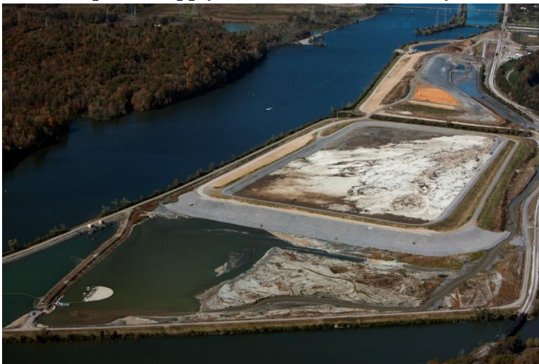
Coal ash waste ponds at the Bull Run Fossil Plant near Clinton, TN, run up against the Clinch River and the north bank of Bull Run Creek.
