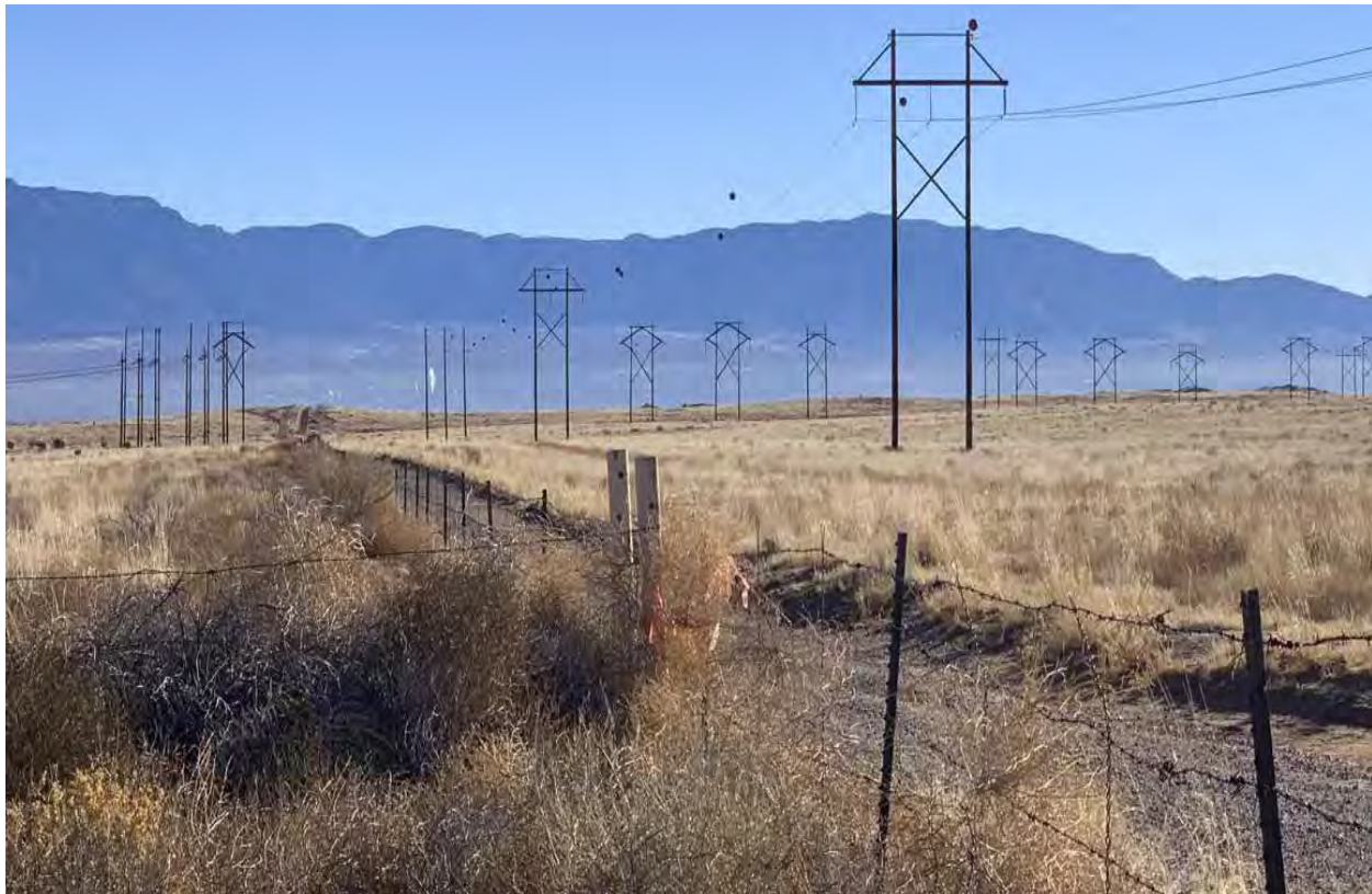
Figure 4: Available Electrical Services
